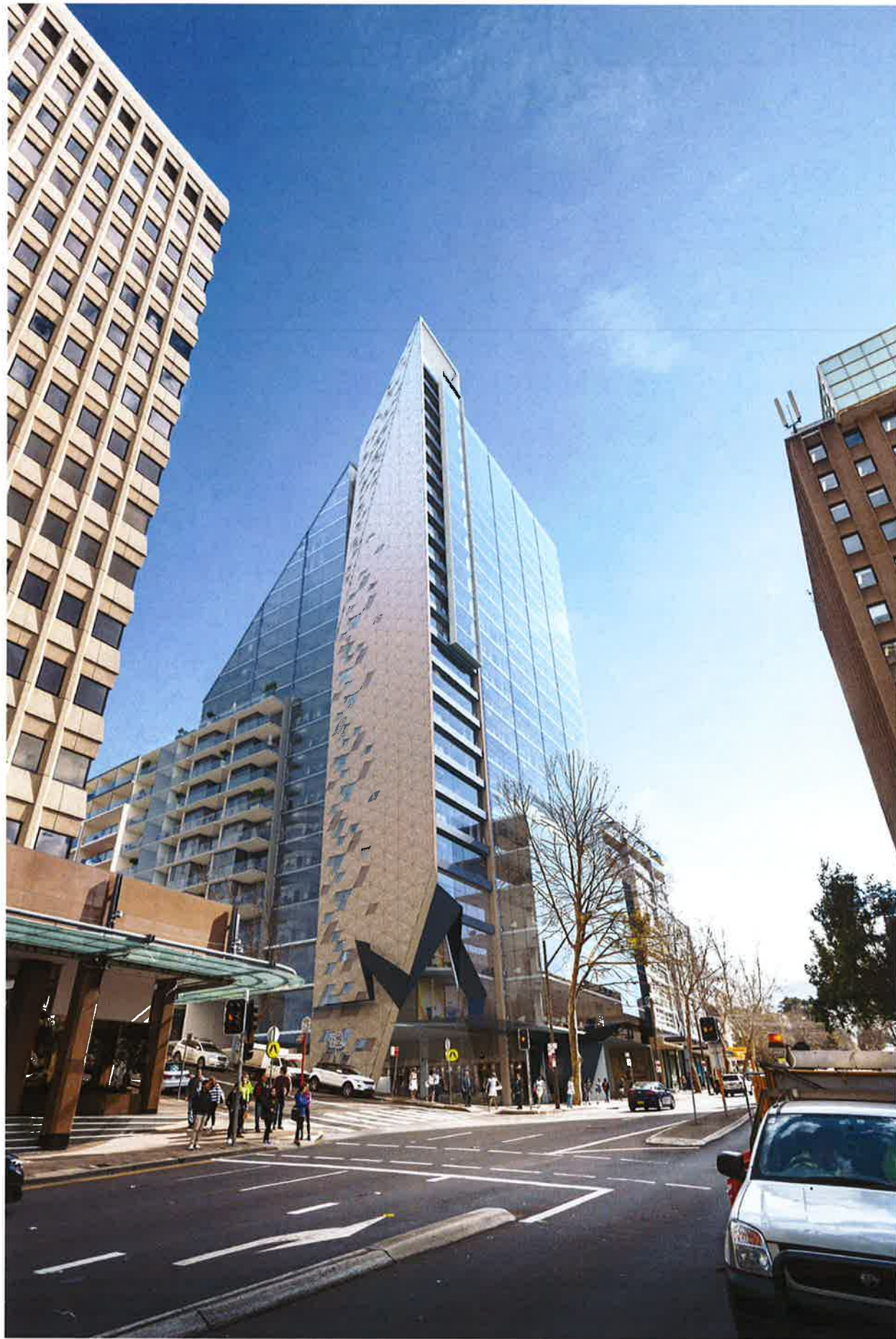
CORNER OF PACIFIC HIGHWAY & BERRY ST
